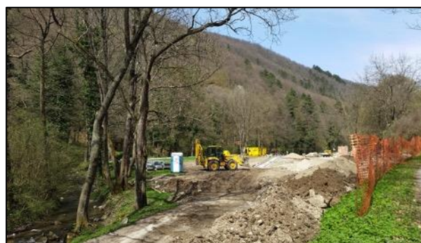
(b) Construction of Dubok Campground at Papuk NP
