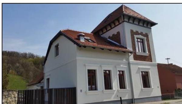
(a) Renovated Administration Building of Papuk NP
